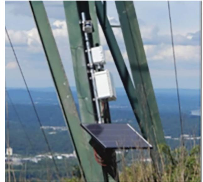
*LineVision system as deployed in the field*
