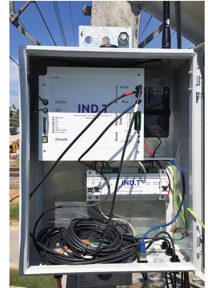
*EFD capacitive coupling sensor mounted on a steel lattice tower to monitor a 138kV conductor (left); and IND.T data collection unit affixed to tower leg showing three coaxial cables from up-tower sensors (right)*
