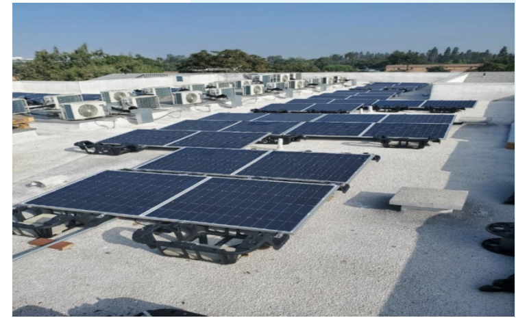
HVAC units and the bi-facial solar array at Willowbrook
