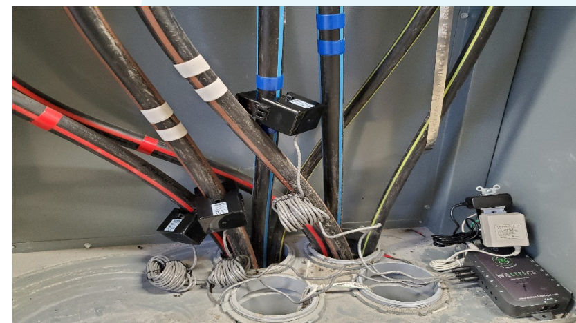
One of the installed Wattrics units monitoring the main incoming power lines using 400A CT's
